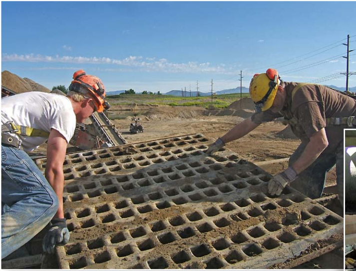
Two workers wrestle to remove a sheet of side-tensioned traditional media.
