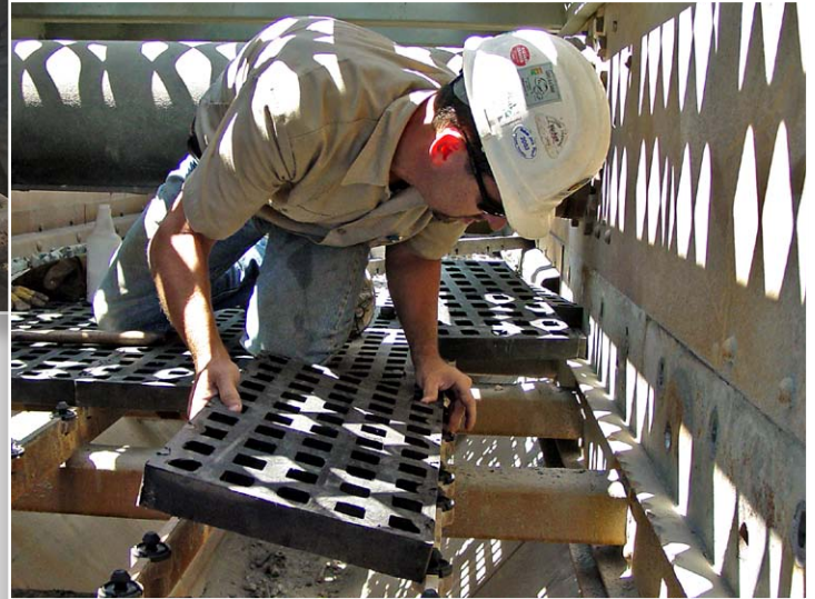
One person can easily install a 1' x 2' Polydeck rubber screen panel, even in the tight confines of a middle deck.
